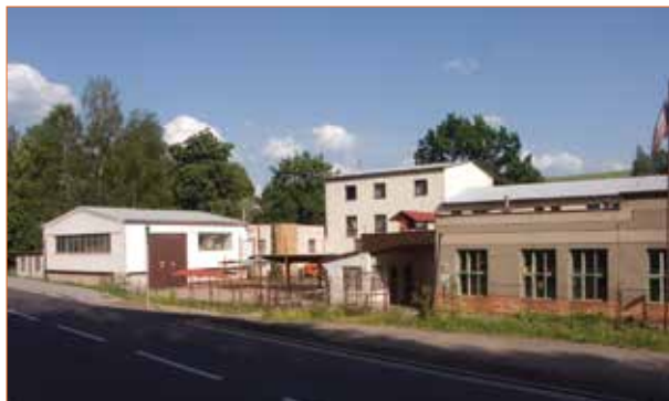
Celkový pohled na budovu školy – uhelna Overall view of school building – coal
