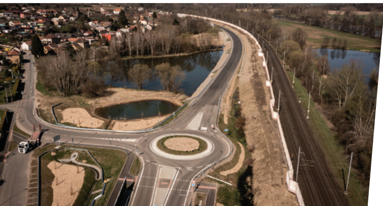
Modernizace silnice II/322 Kojice Modernization of the road II/322 Kojice
